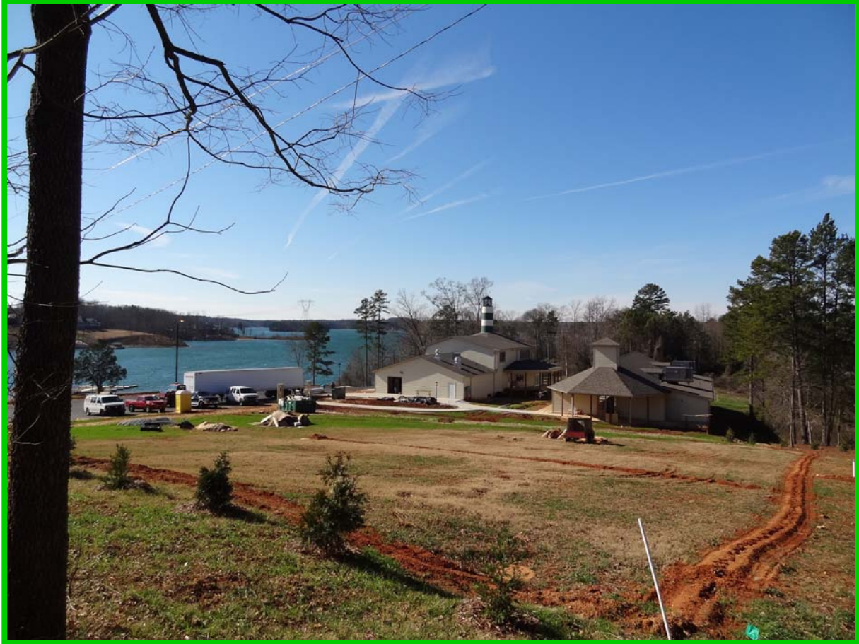
"The Lighthouse takes shape" ©Copyright 2012 Integrity Realty, Inc.
